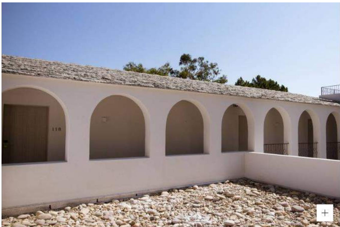
Exterior details Misincu
